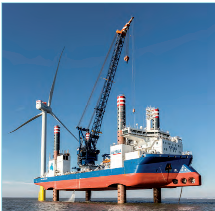
► The vessel The Sea Installer
