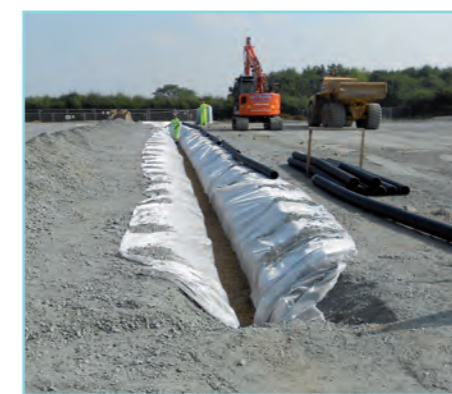
► Site preparation work underway at Necton
