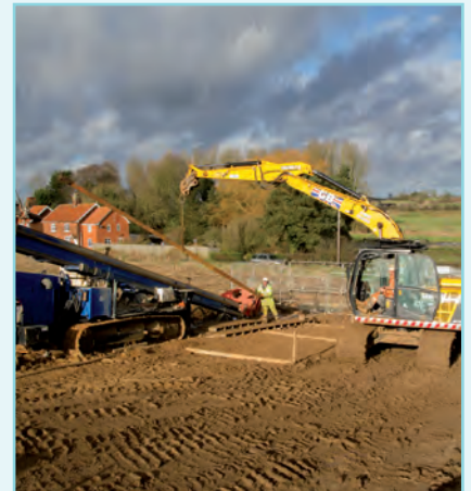
▶ Work on the cable corridor at Great Ryburgh
