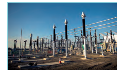
► Substation construction continuing at Necton
