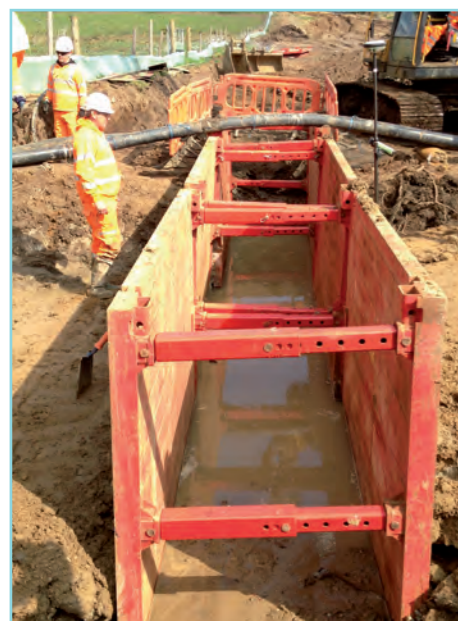
► Installing the onshore cable under the River Stiffkey
