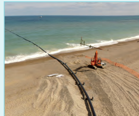
► Export cable ducting pull-out at Weybourne
