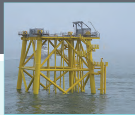
► The offshore substation jacket secured in position
