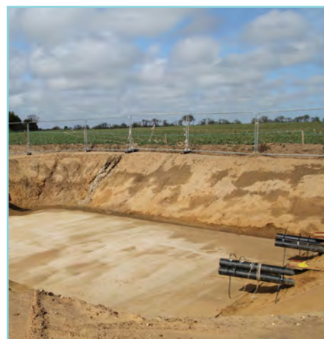
► A joint bay being constructed
