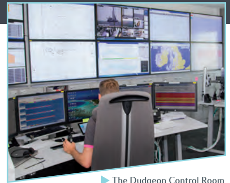
▶ The Dudgeon Control Room
