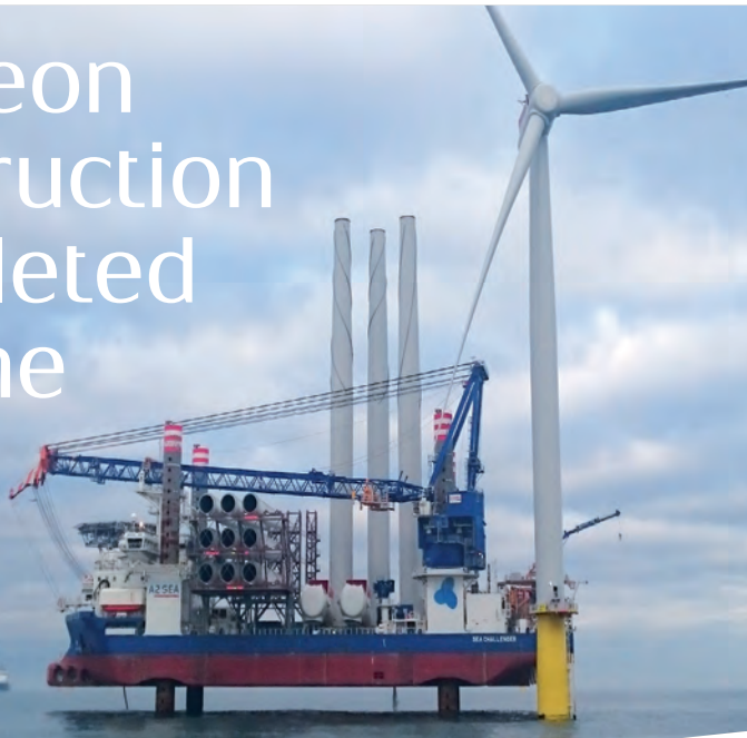
▶ Sea Challenger from A2Sea installed Dudgeon's 67 wind turbine generators
